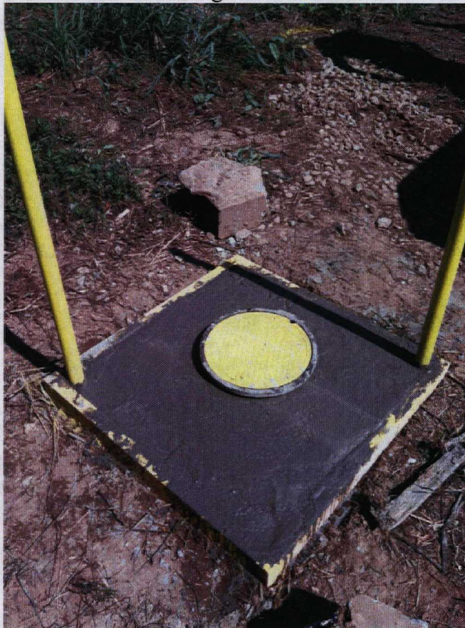
Monitoring well 2D being repaired.
