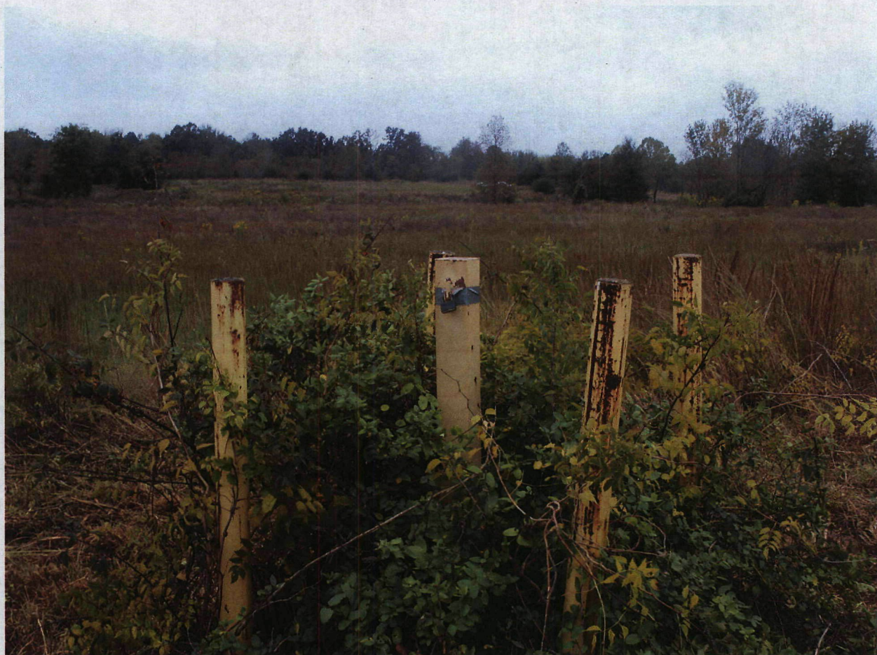
Photo 17: Well MW-109, overgrown.
