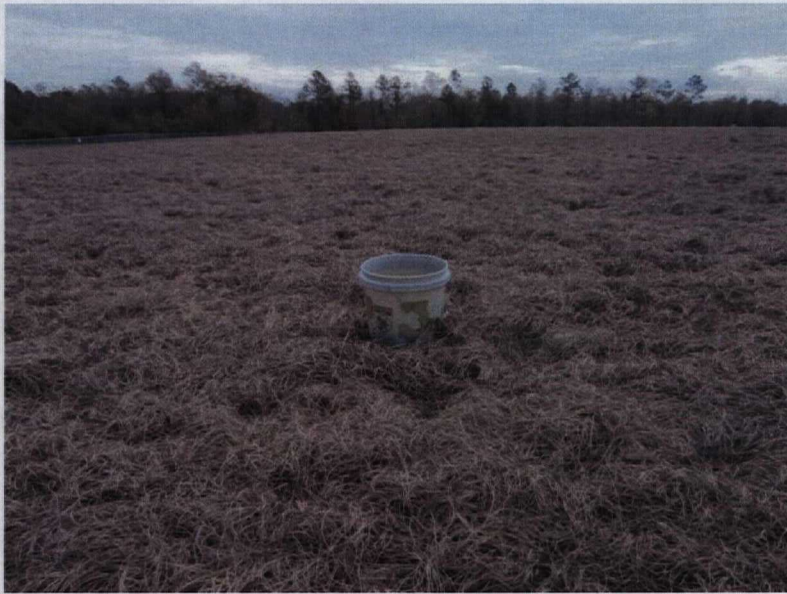
View of vegetative cover on cell and one of four settlement markers.
