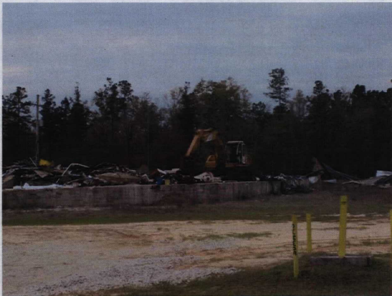
Scrap metal operations on the slab of the former one-story building.
