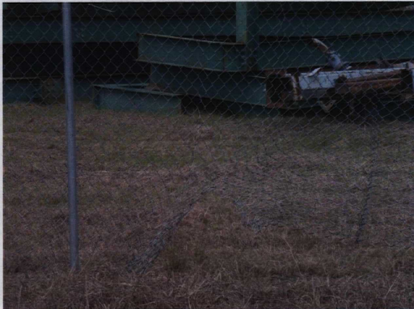
Small damaged section of fence that surrounds the capped area.
