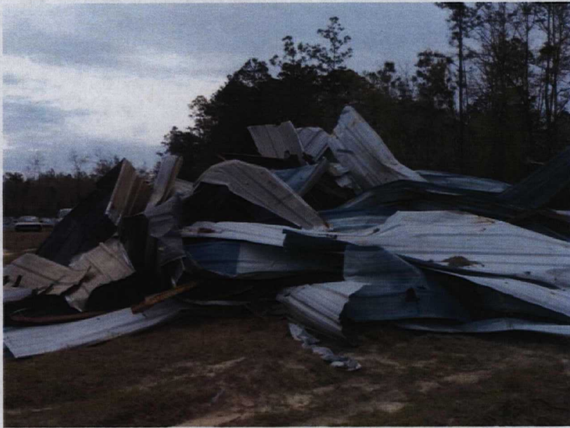
Scrap metal located in southwest corner of the Site.
