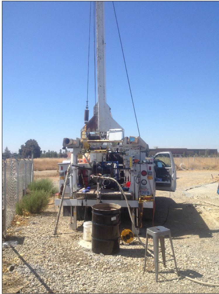
Development rig setup on MW-4C-R.
