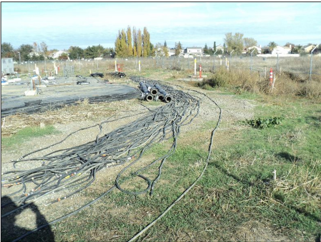
Wires and manifolds staged off cap.
