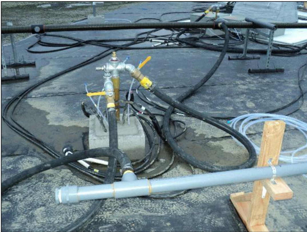
Wellhead installed, wires connected, and vacuum extraction lines (VEUs) connected to manifolds.
