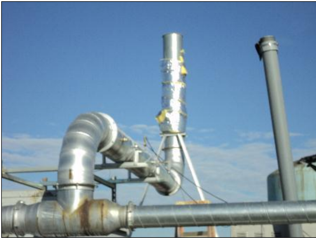
Discharge stack for multiple blower operation.
