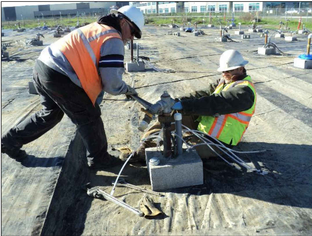
Removal of wellhead.
