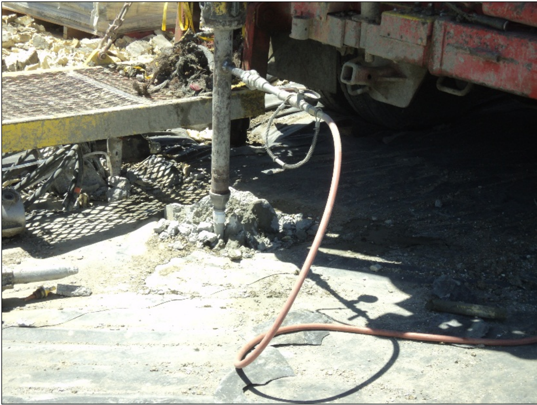
Pressure grout at a wellhead.
