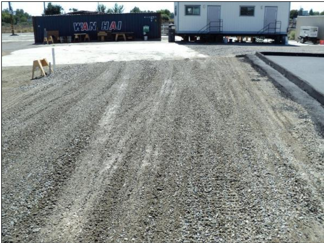
Rock pad placed next to treatment pad for use with power supplies. Office trailer in background.
