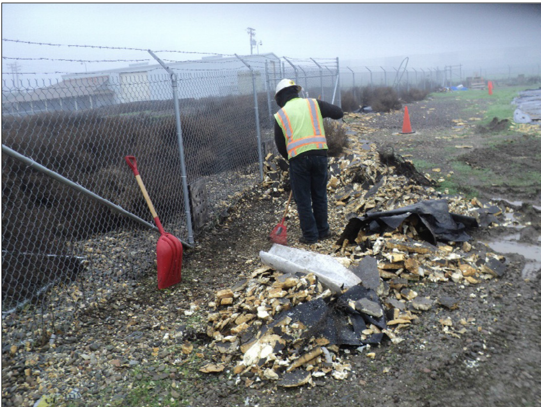
Collection of stray cap insulation around the site.
