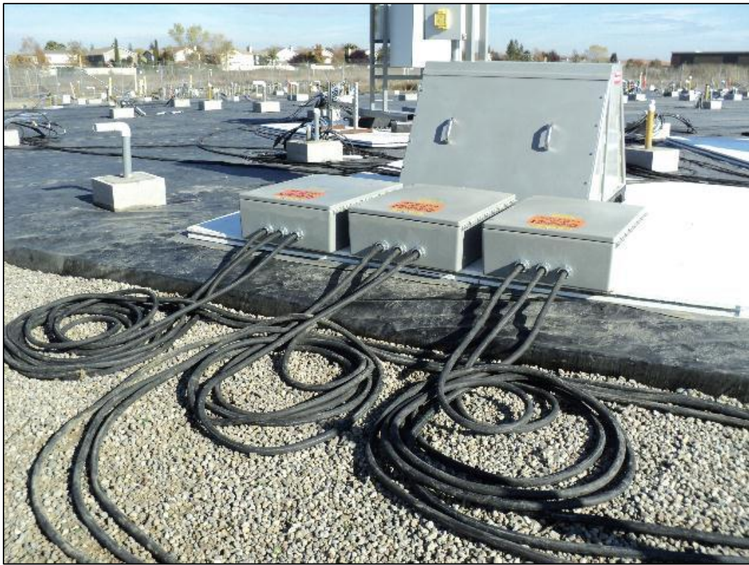
Wires placed on cap.
