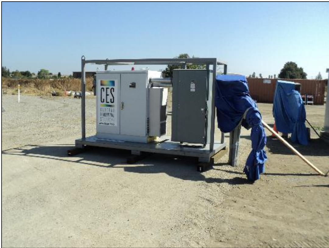
Power supply delivered and placed at site (awaiting electrical connections).
