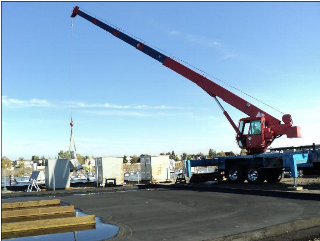
Placement of current transducer.
