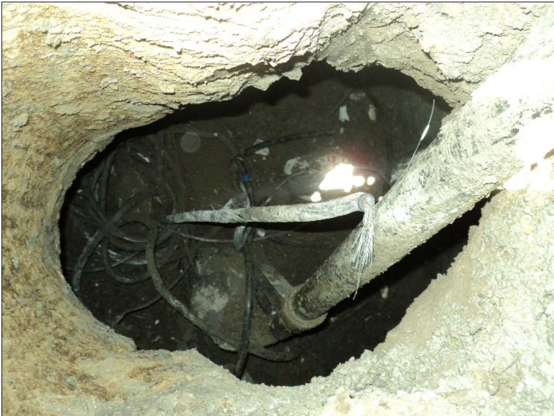
Void found at electrode F2.
