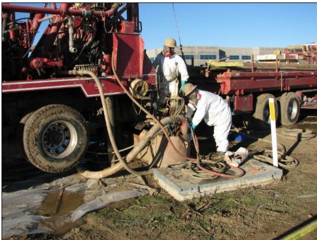
Full-face respirators during installation of Preliminary Monitoring Points (PMPs). 2008.
