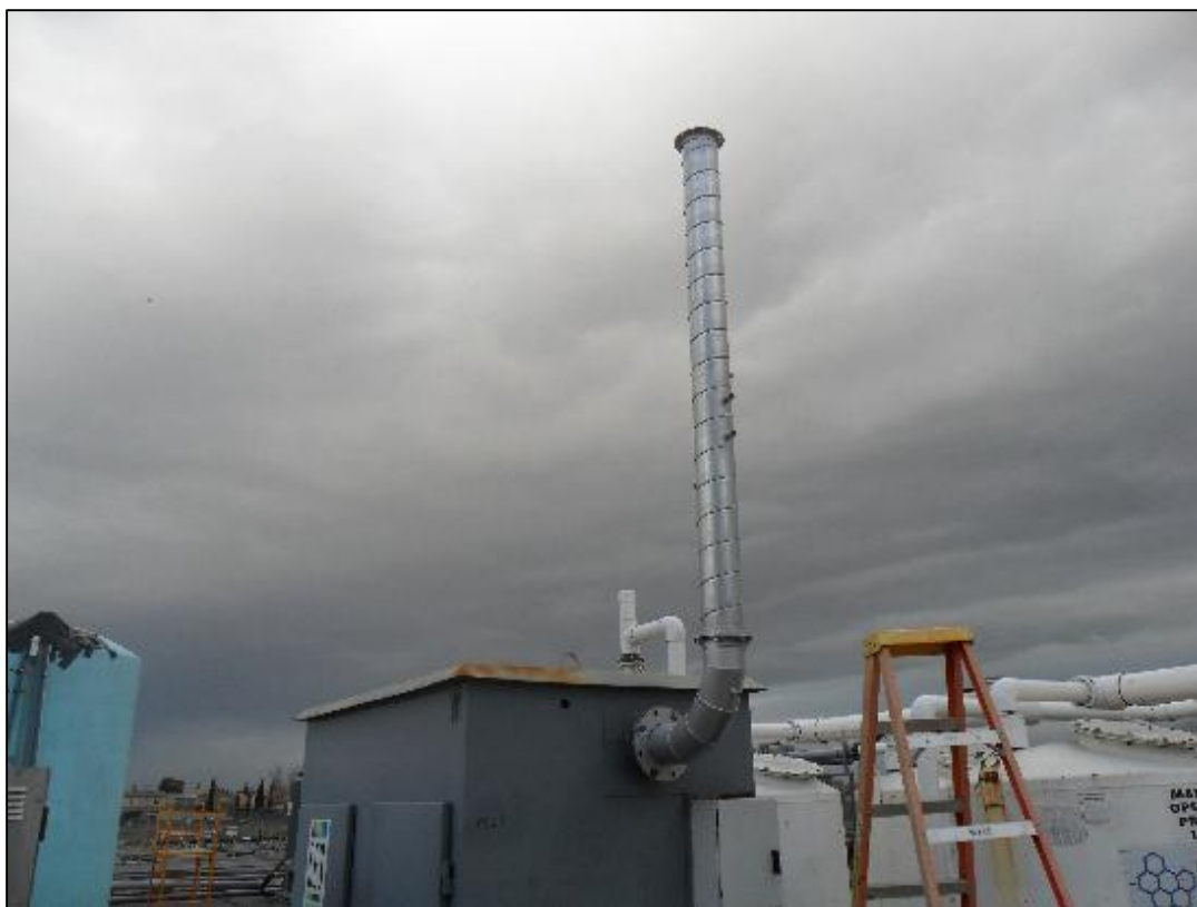
Discharge stack (for startup and Stage 1 with only single blower operation).
