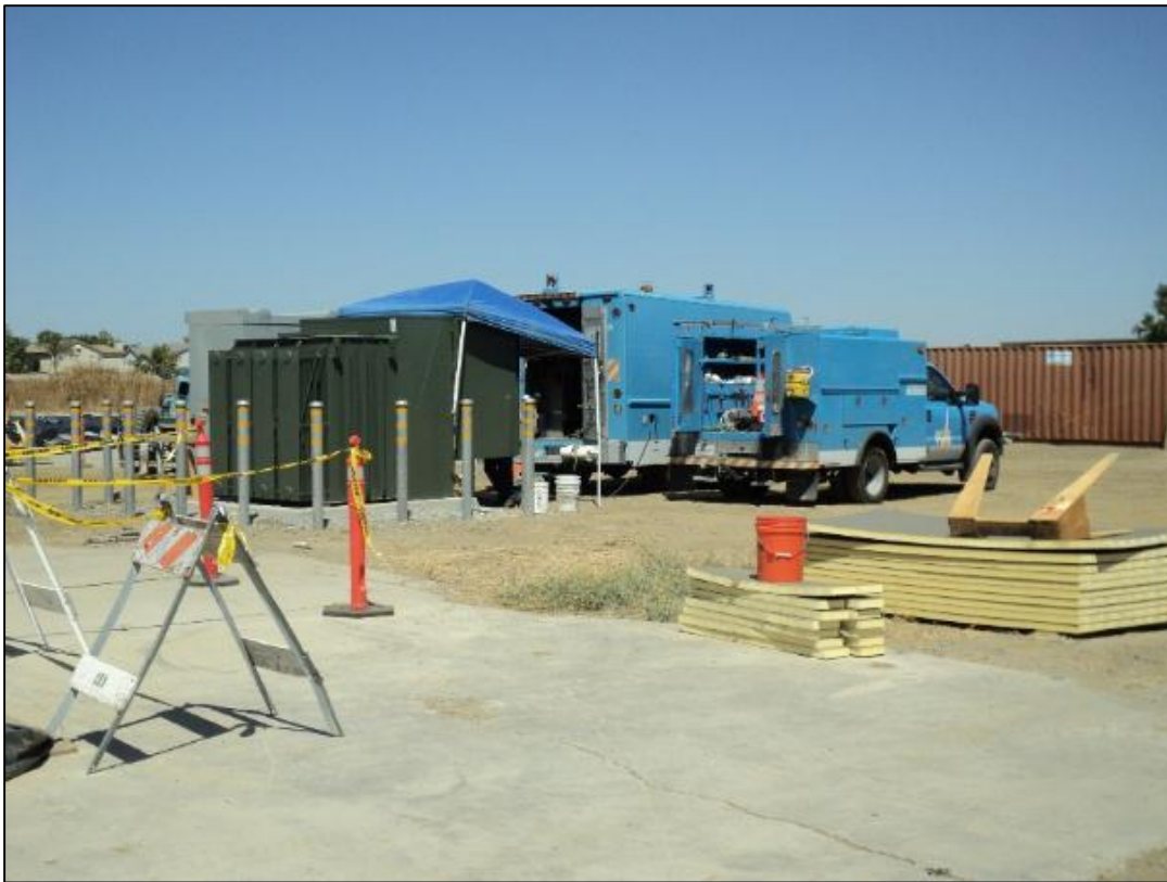
PG&E working on transformer.
