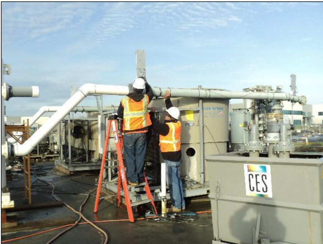
Additional equipment removal.
