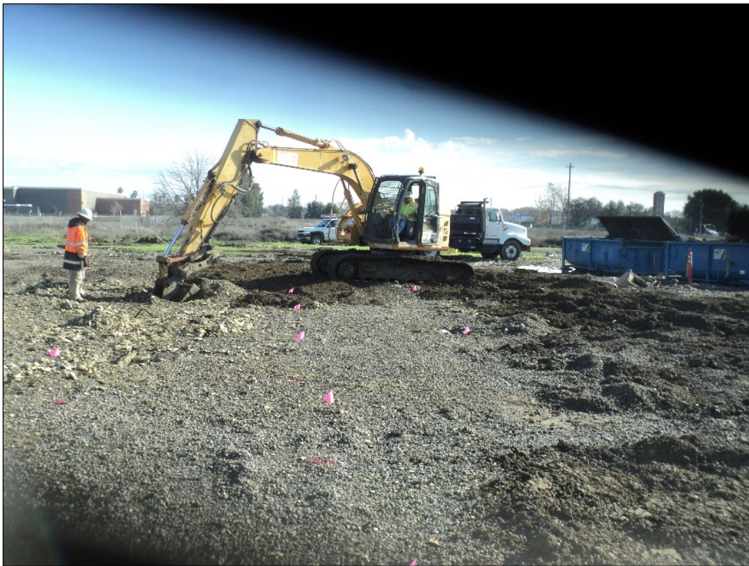
Excavation of puppy electrodes. Pink flags denote location of puppy electrodes (Note: camera was undergoing failure of automatic opening lens cover).
