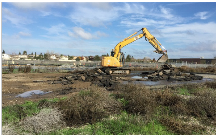
Breakup of the asphalt treatment pad.
