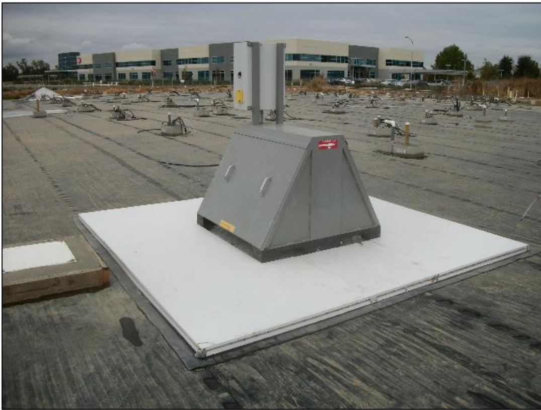
Placed current transformer.
