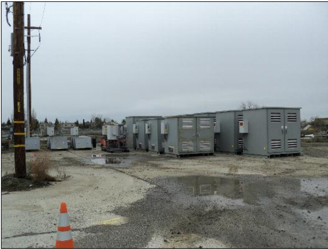
Equipment staged for loading.
