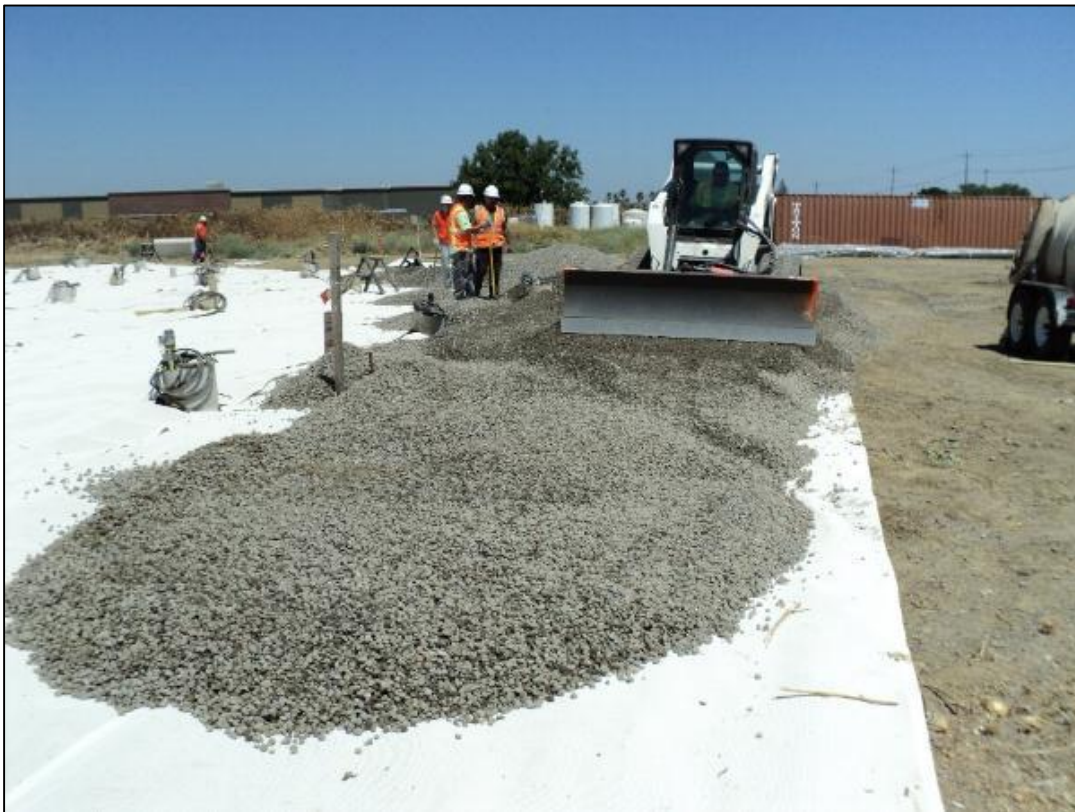
Placement of gravel layer on cap screen.
