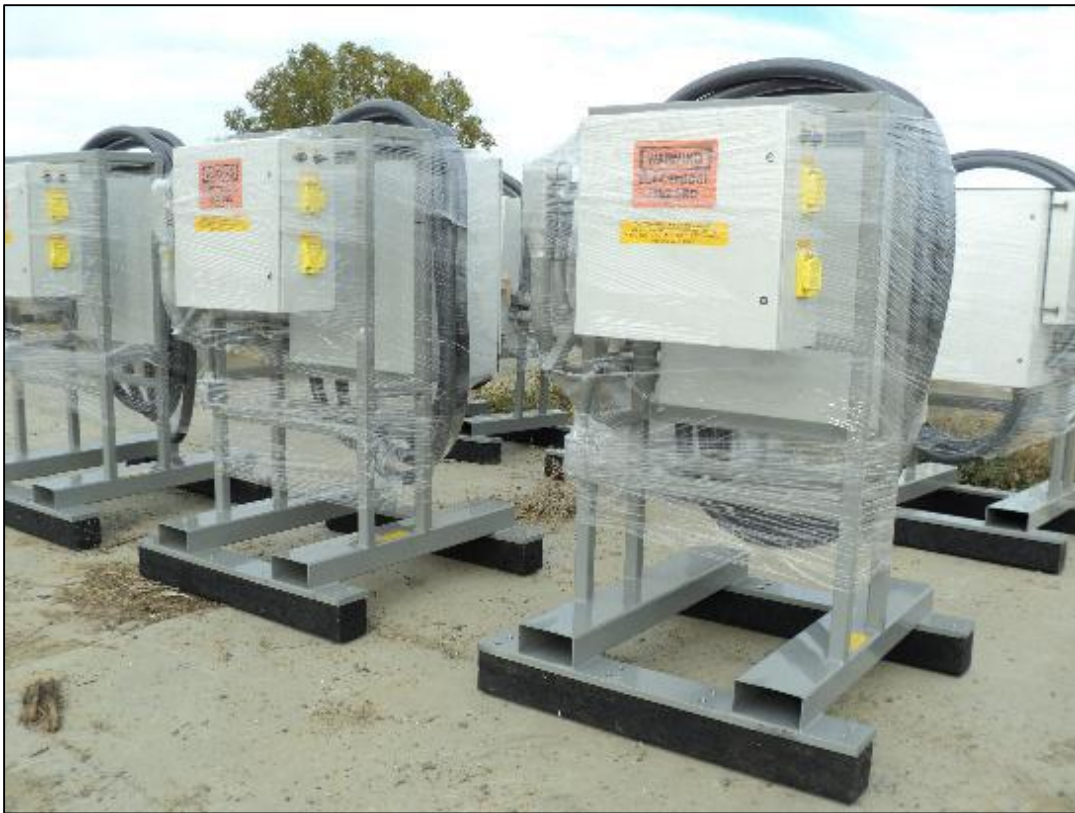
Delivered drip skids.
