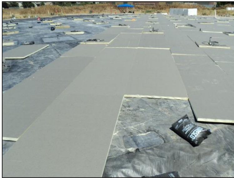
Placement of insulation board onto cap.
