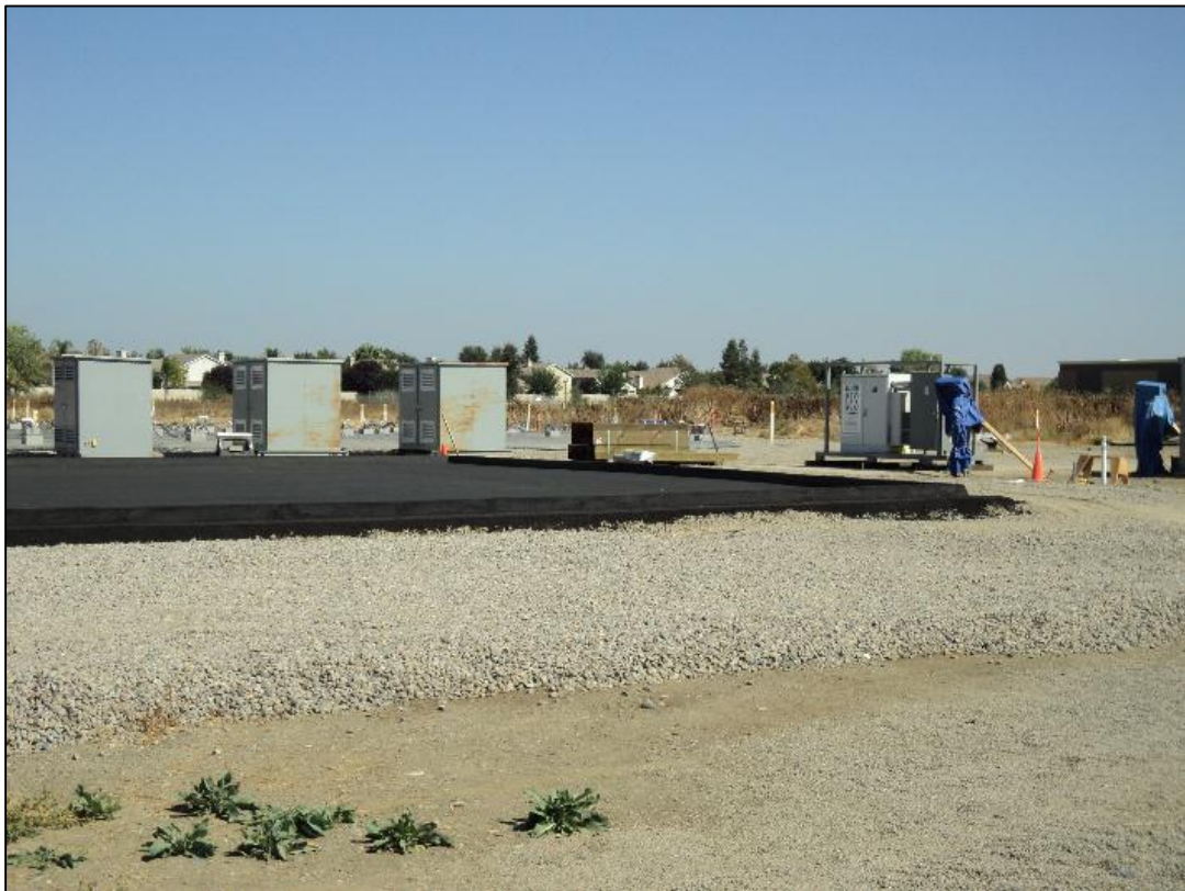
Three transformers and a power supply; treatment pad in foreground.
