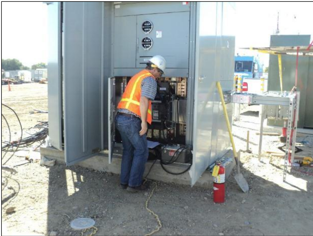
Switchgear testing in progress.
