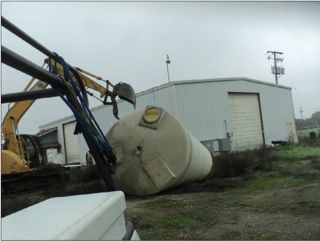
Moving the 6,500-gallon tank into position to be later cut into pieces prior to disposal.
