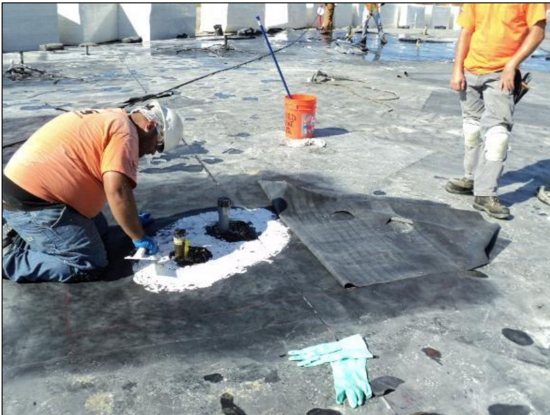
Sealing cap penetrations.
