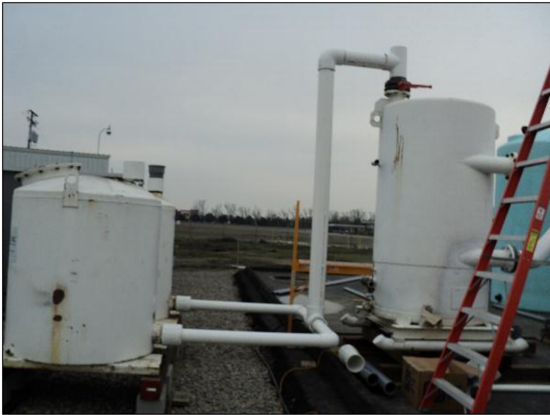
Plumbing from coalescer to vapor phase carbon units.
