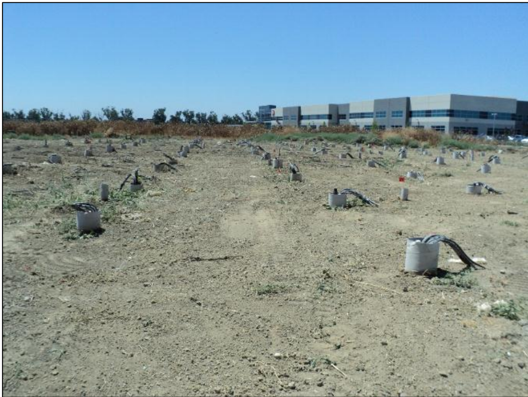
Field ready for cap install. 2010.
