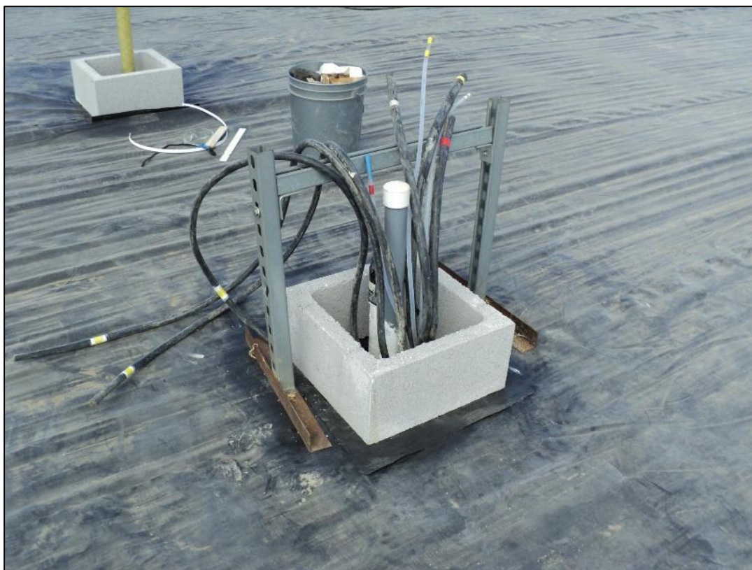
Wellheads prepared for grout.
