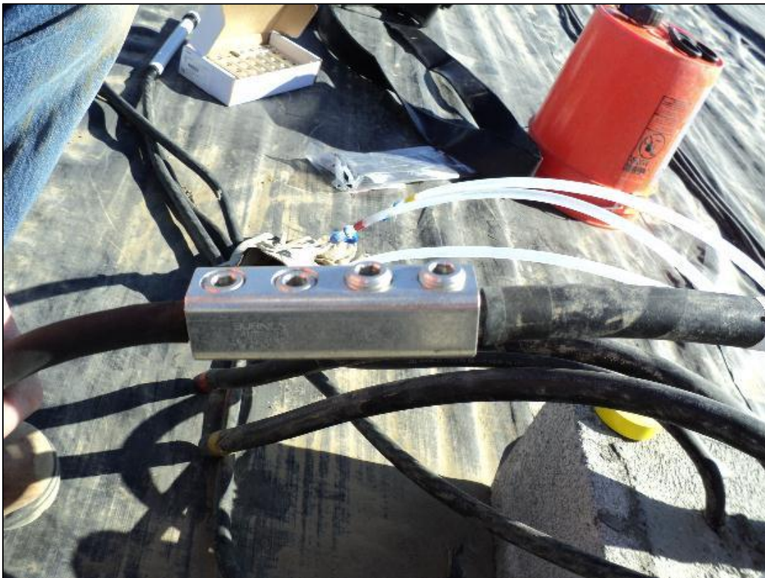
Connecting wires, in progress.
