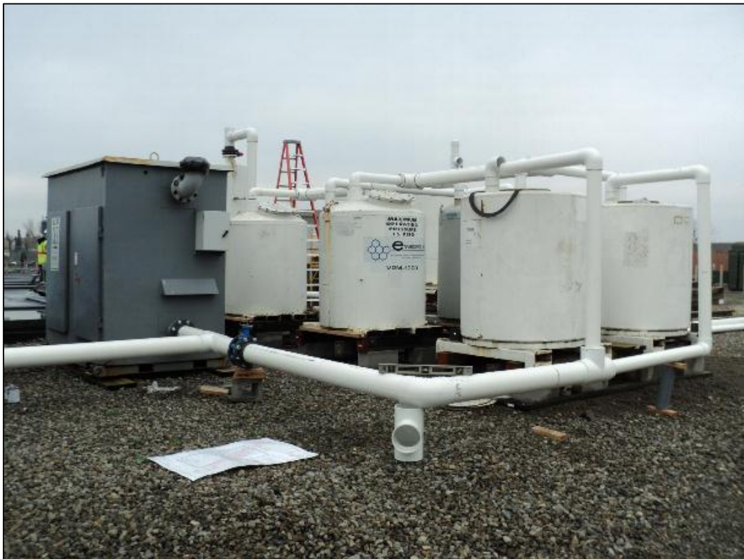
Granular activated carbon (GAC) vessels.
