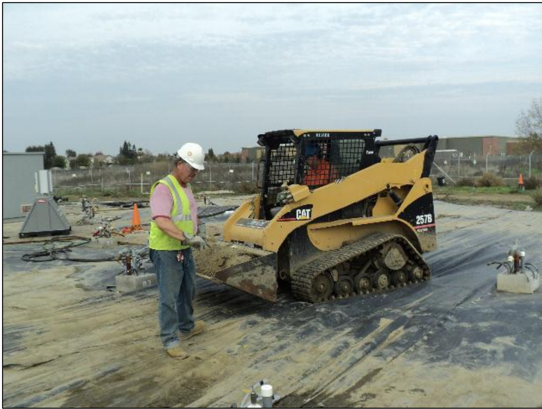
Cleaning cap sediments released from manifold.
