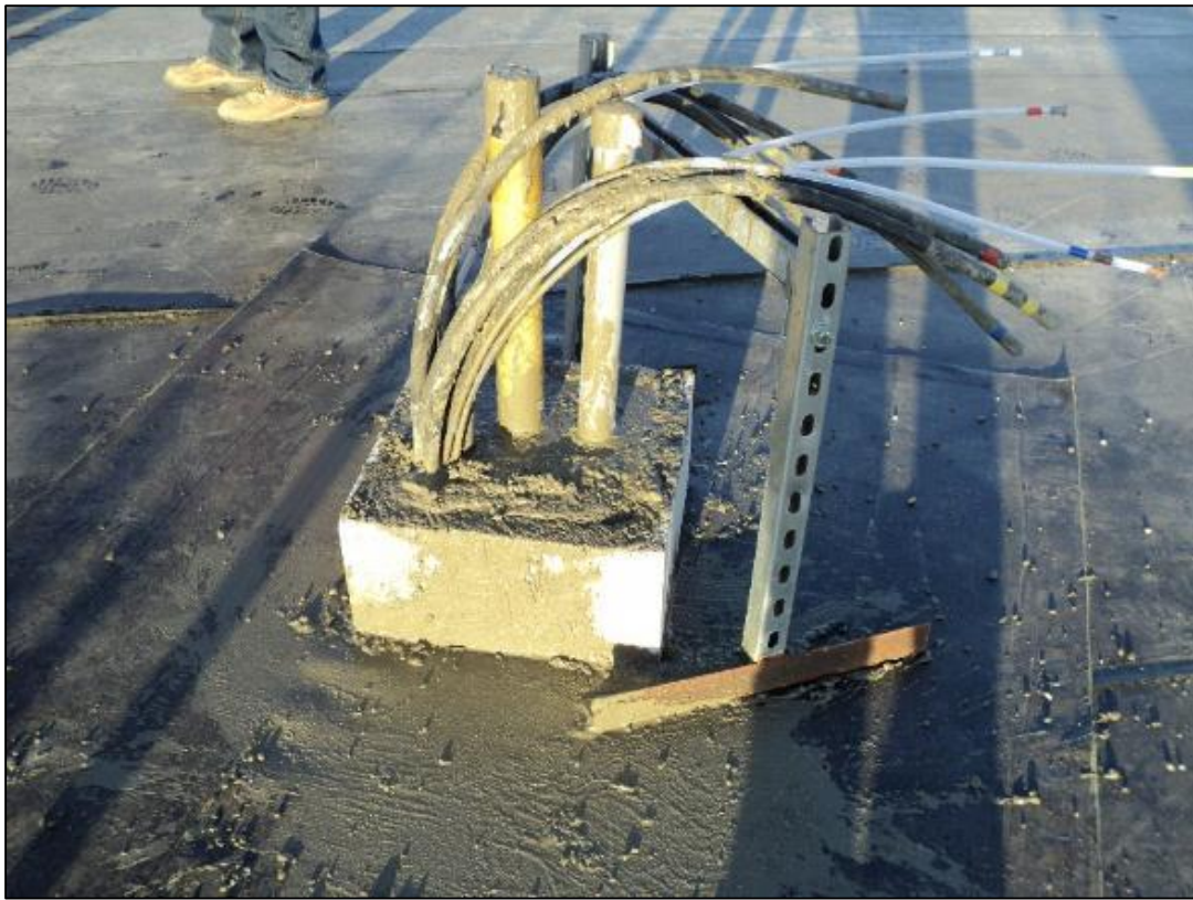
Grouted wellhead.
