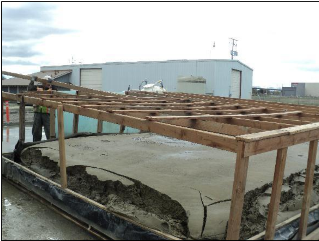
Sediments removed, separated, and dewatered during treatment (vapor-containing cap removed).
