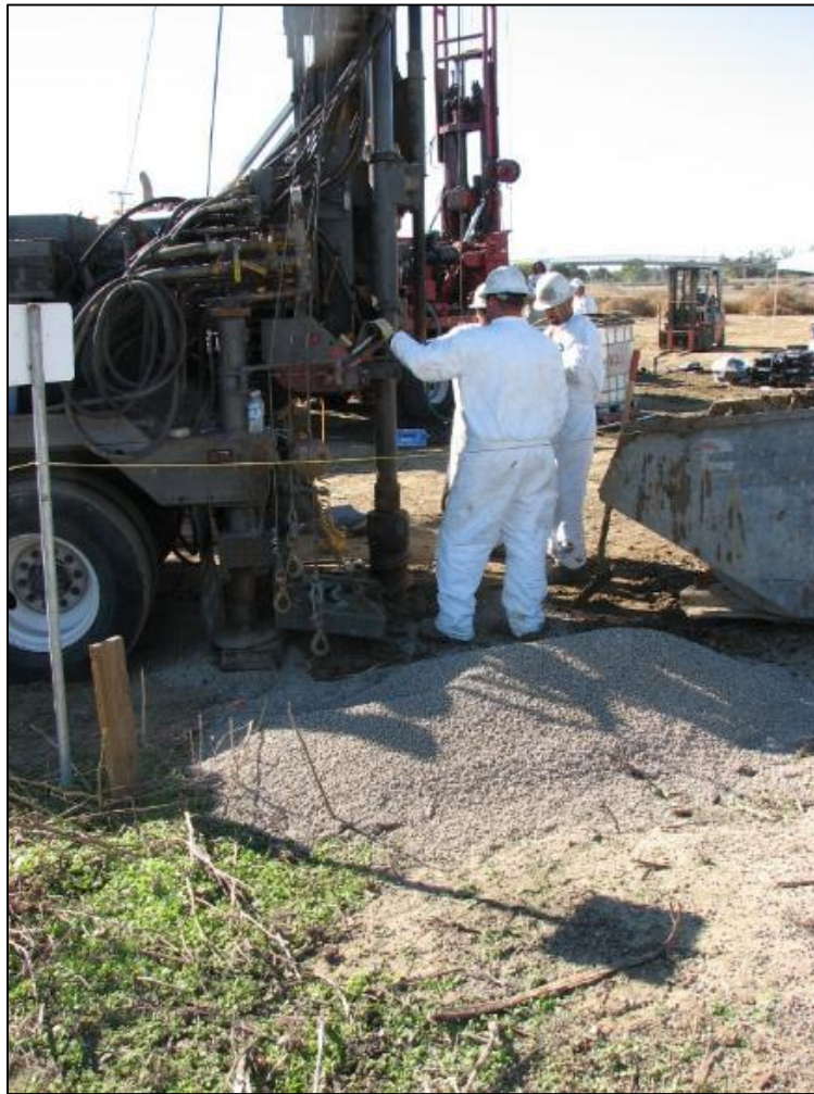
Installation of electrodes; temperature monitoring wells (TMWs). 2009.
