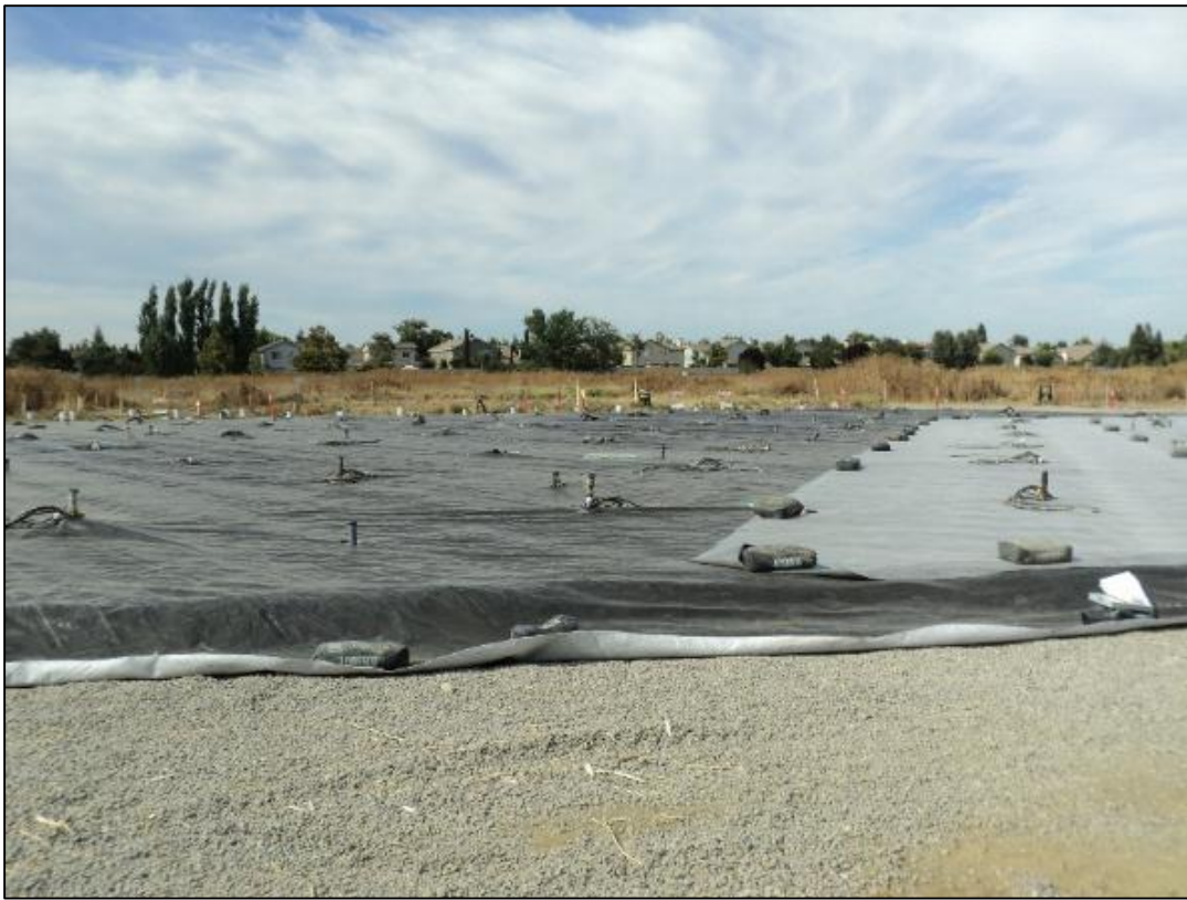
Layer of EPDM (right side) over layer of high-density polyethylene (HDPE).
