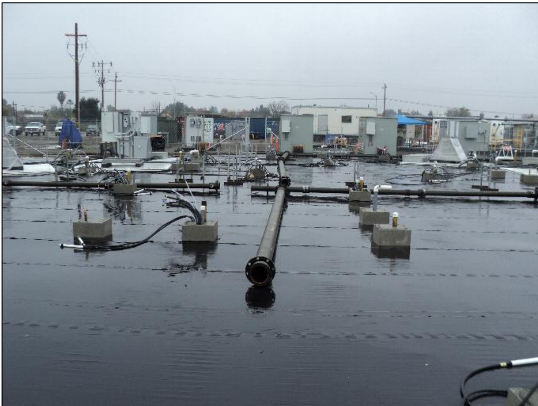
Placement of the vapor extraction manifold.
