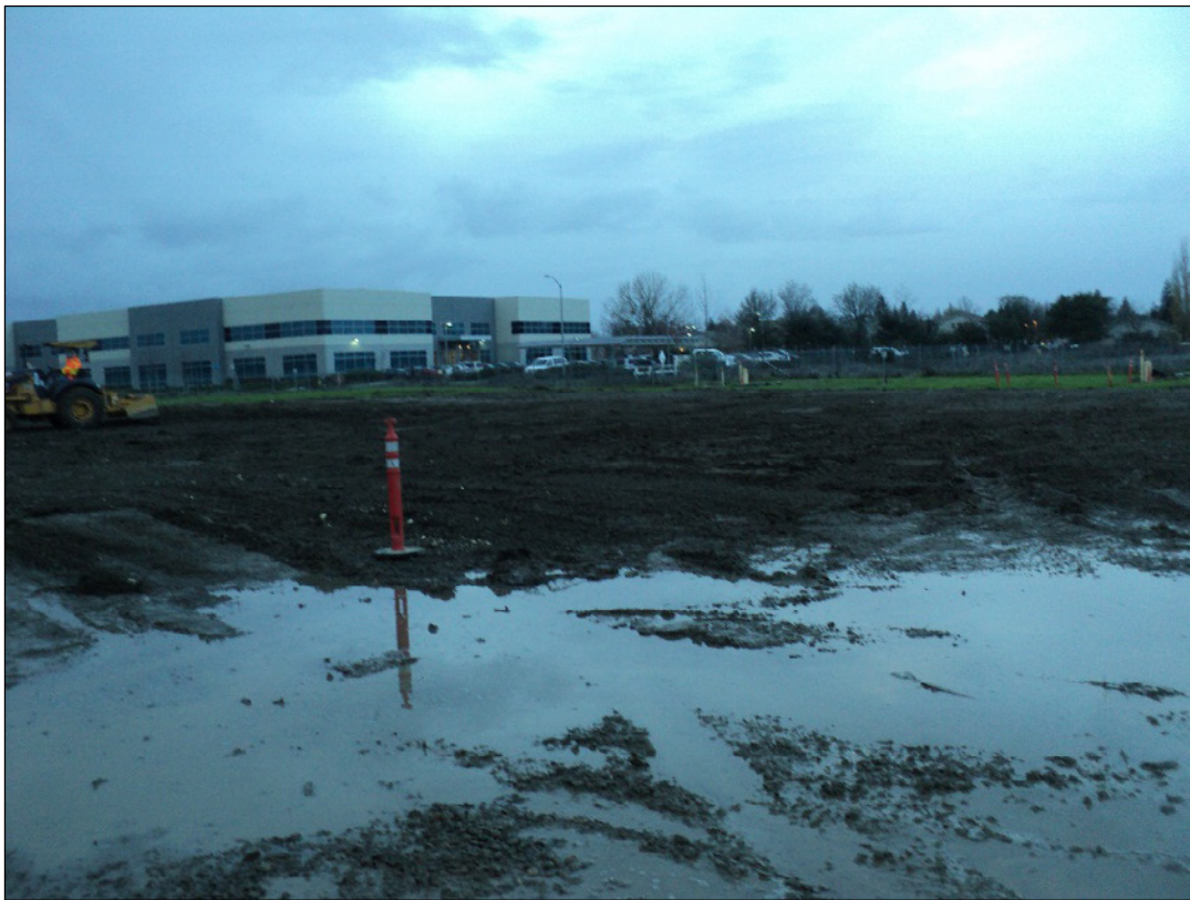
Final site grading.
