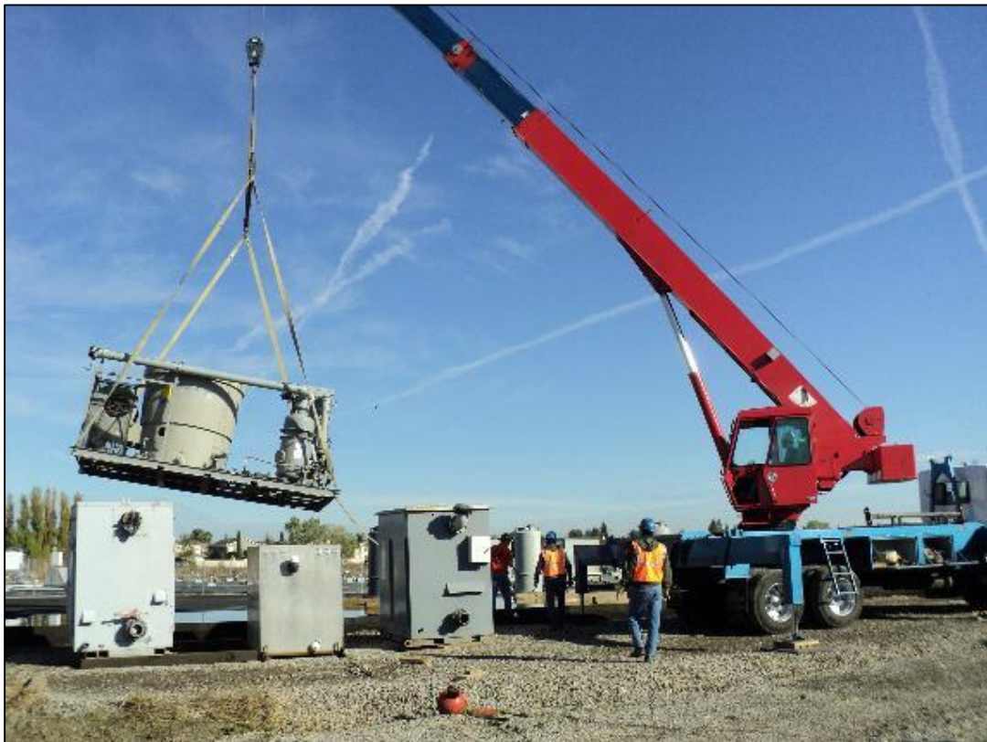
Placement of cooling tower.
