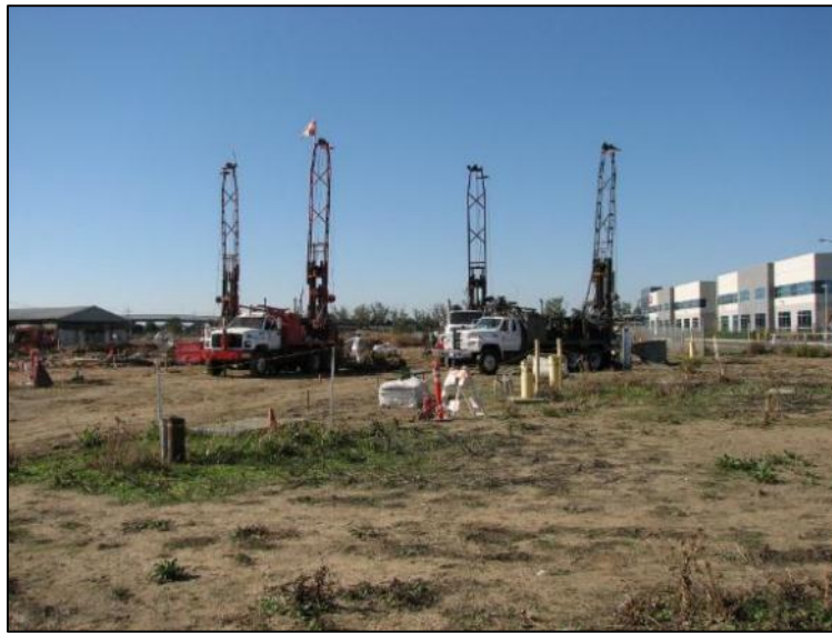
Installation of electrodes; temperature monitoring wells (TMWs). 2009.
