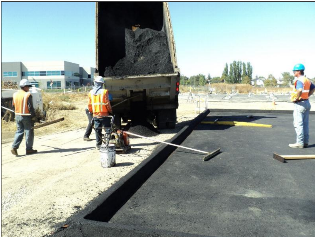
Berm on asphalt pad has been constructed; forklift ramp being installed.
