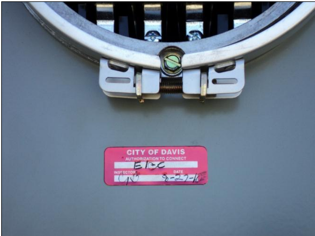
City-approved power for connection.
