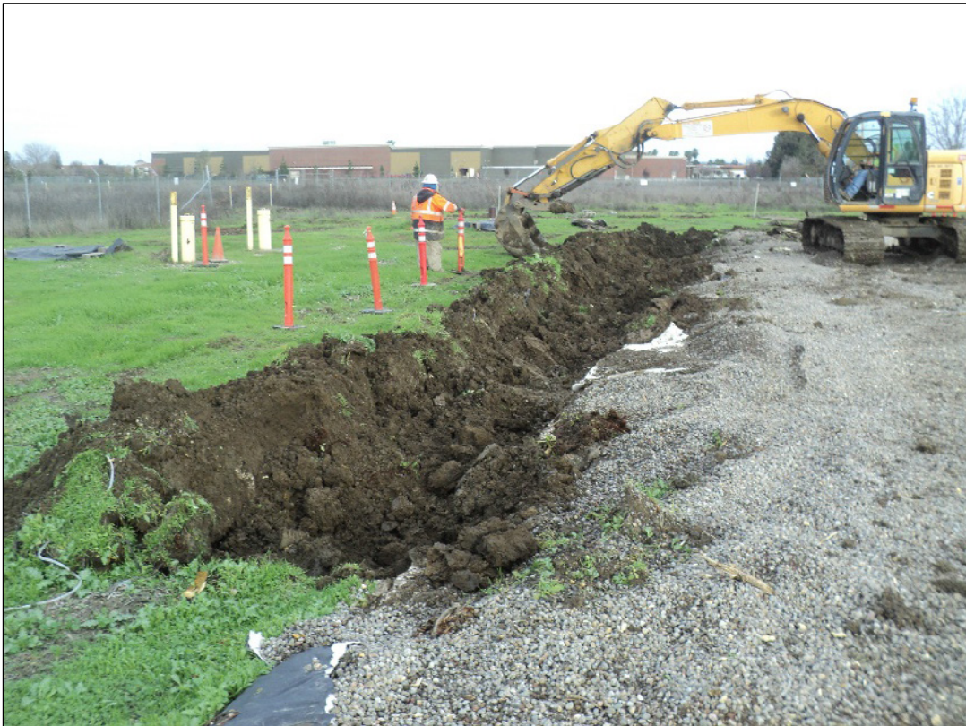
Excavation of buried cap material around perimeter.
