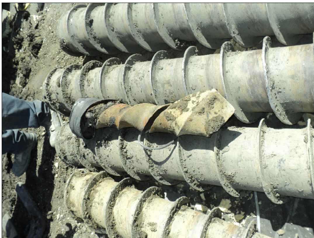
Twisted electrode segment removed from boring.
