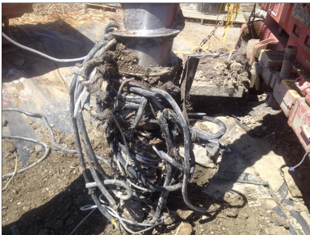
Electrode cables wrapped around auger.
