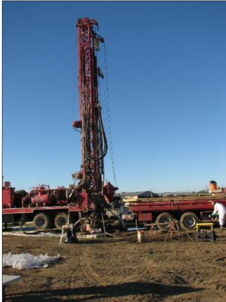
Drill rig and support rig used for installation of Preliminary Monitoring Points (PMPs). 2008.
