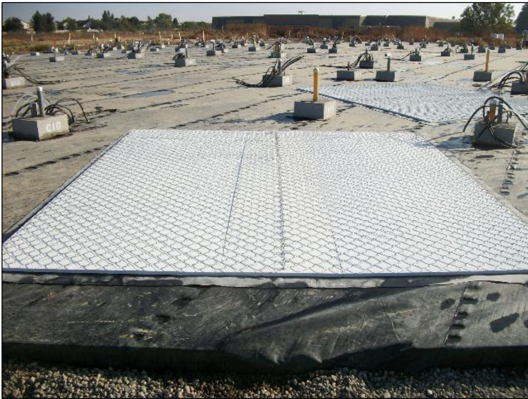
Grounding mats on treatment pad; will be used for current transducers or drip skids.
