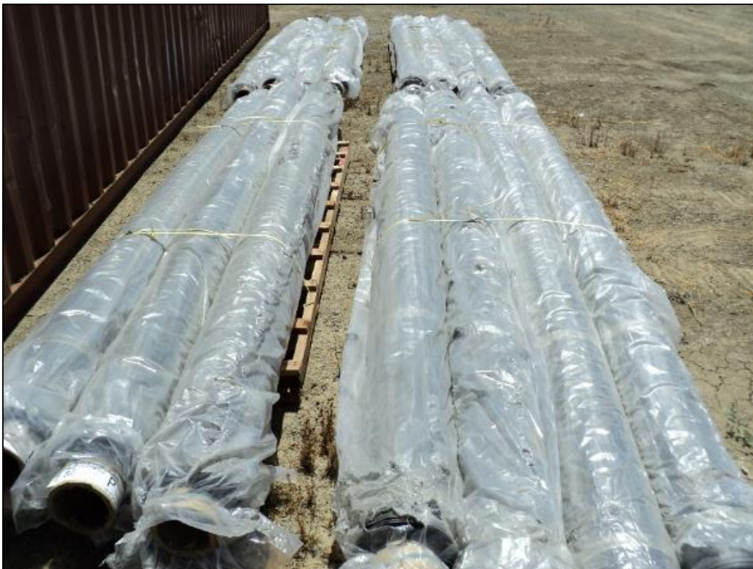
Delivered cap materials. 2010.
