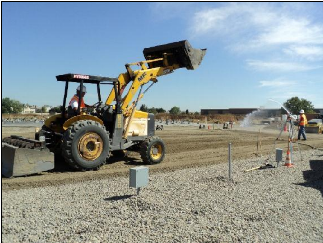
Compacting base for treatment pad.
