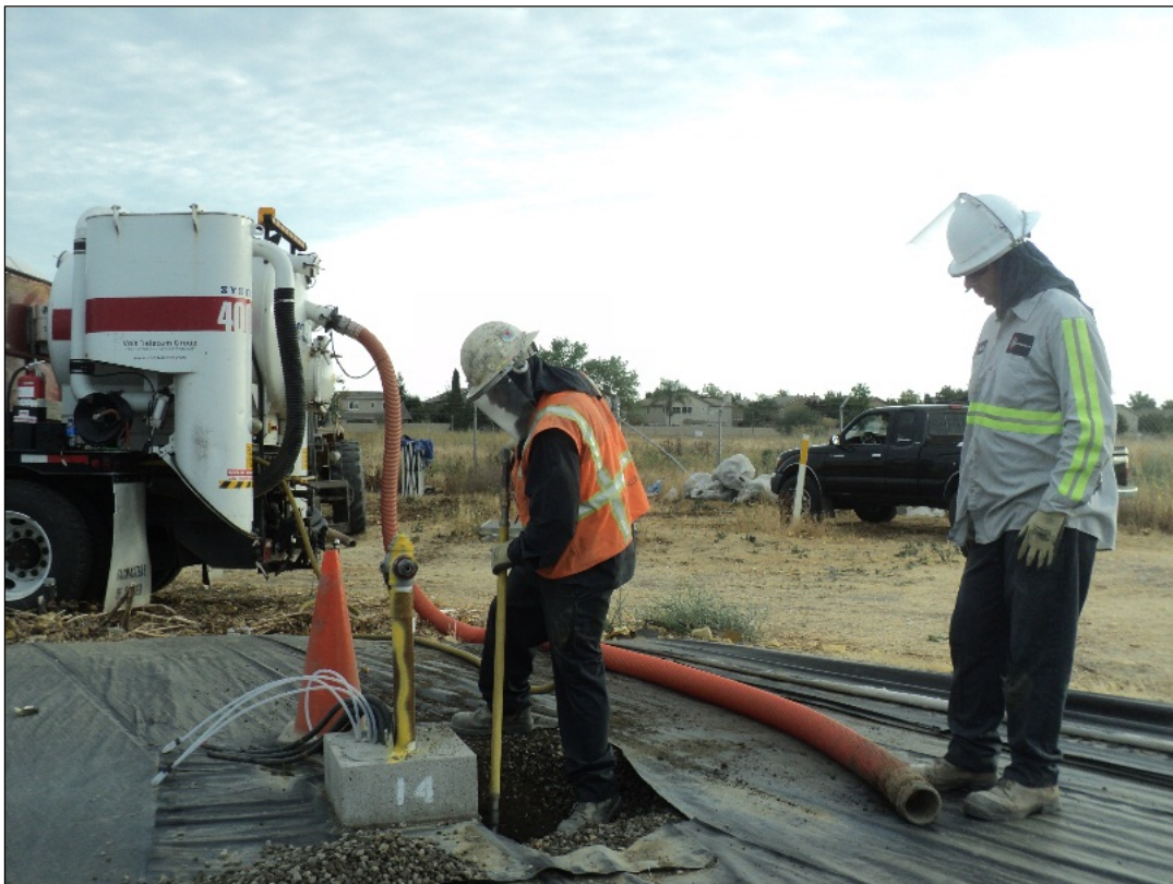
Vacuum truck excavation at wellheads to search for additional voids.
