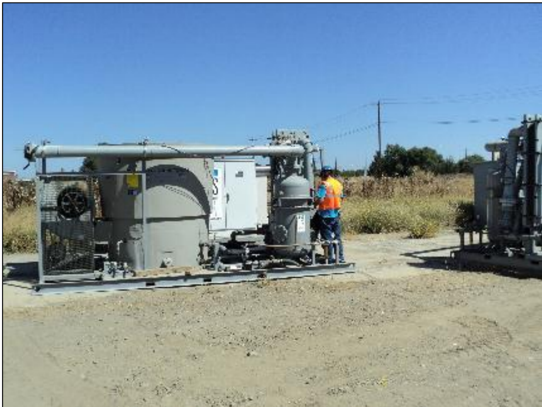
Delivered cooling tower skid.
