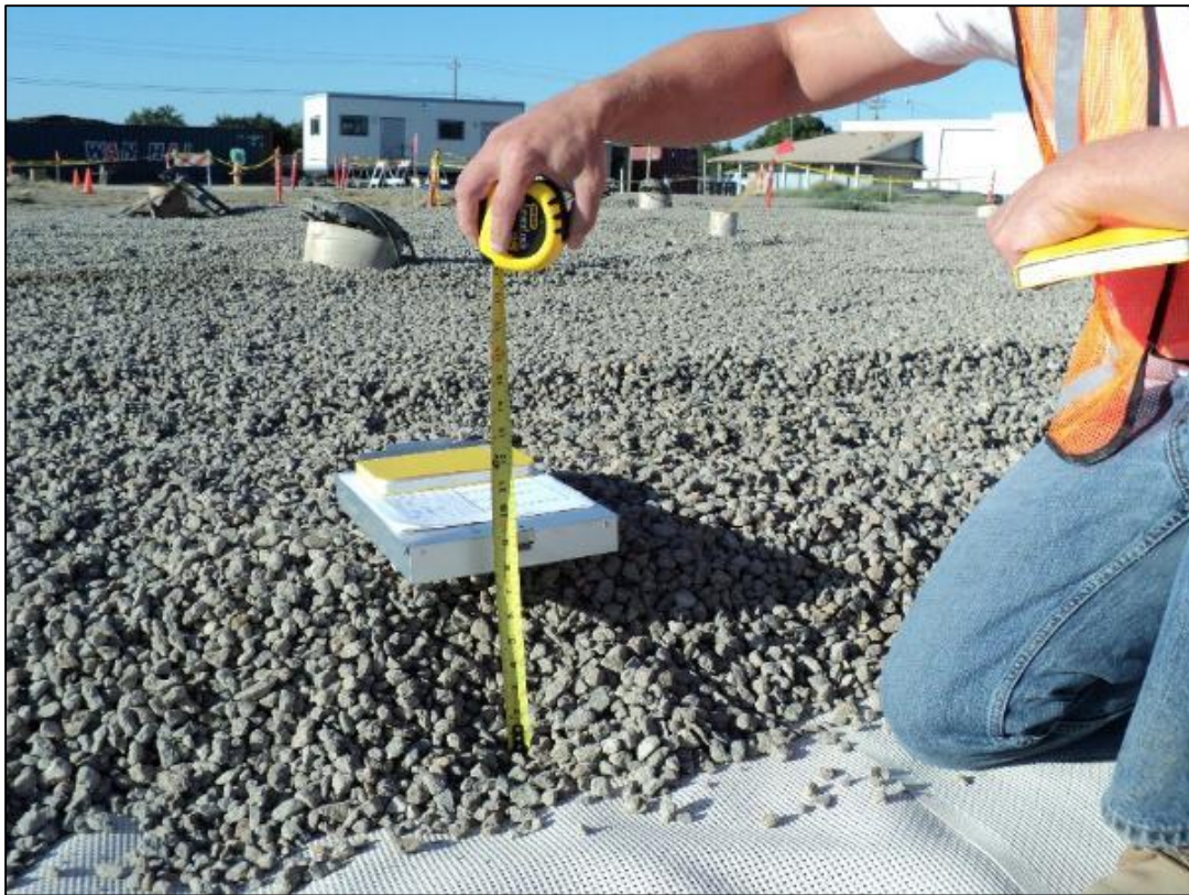
Measuring gravel layer under fugitive emission cap.
