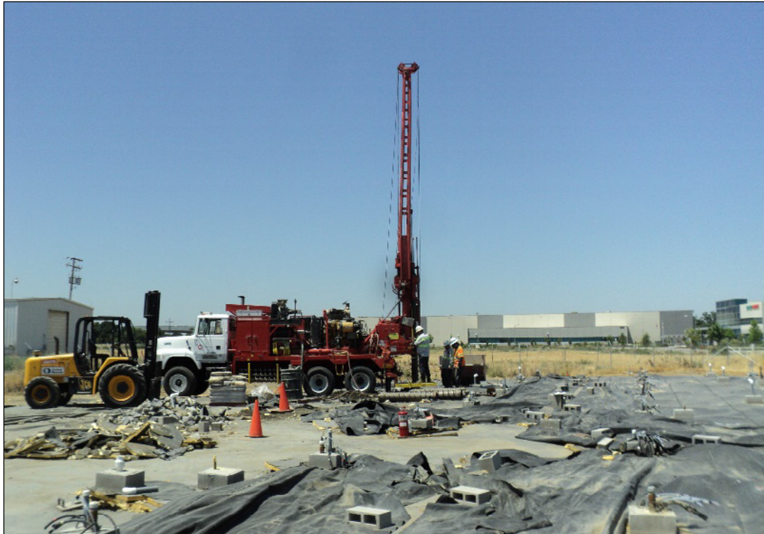
Hollow stem auger rig for electrode and well overdrilling.
