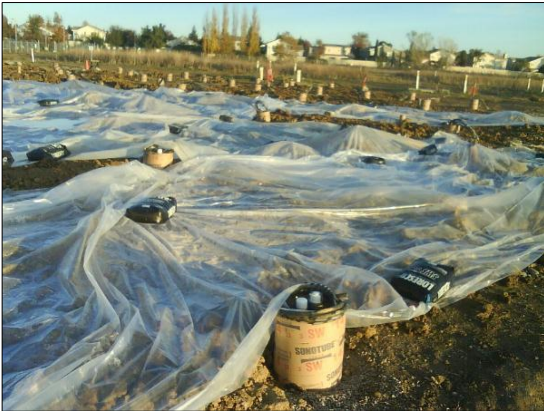
Field after installation. Wellheads protected in tubes awaiting cap installation. Soil cuttings were spread over the shallow treatment areas; these are shown covered in plastic awaiting cap install. 2009.
