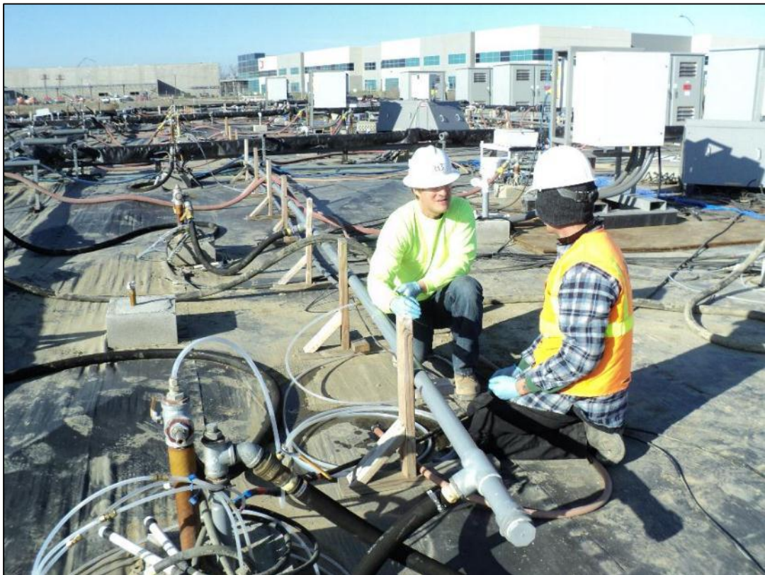
Connecting wells to manifolds.
