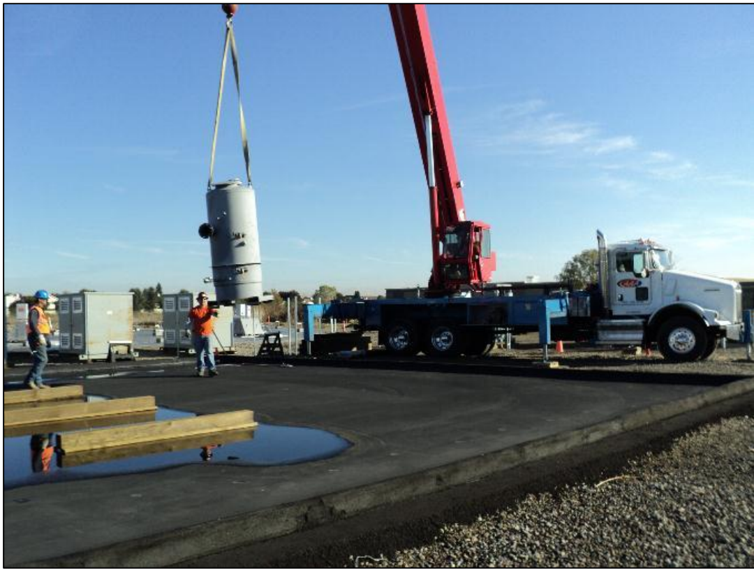
Placement of air/water separator.
