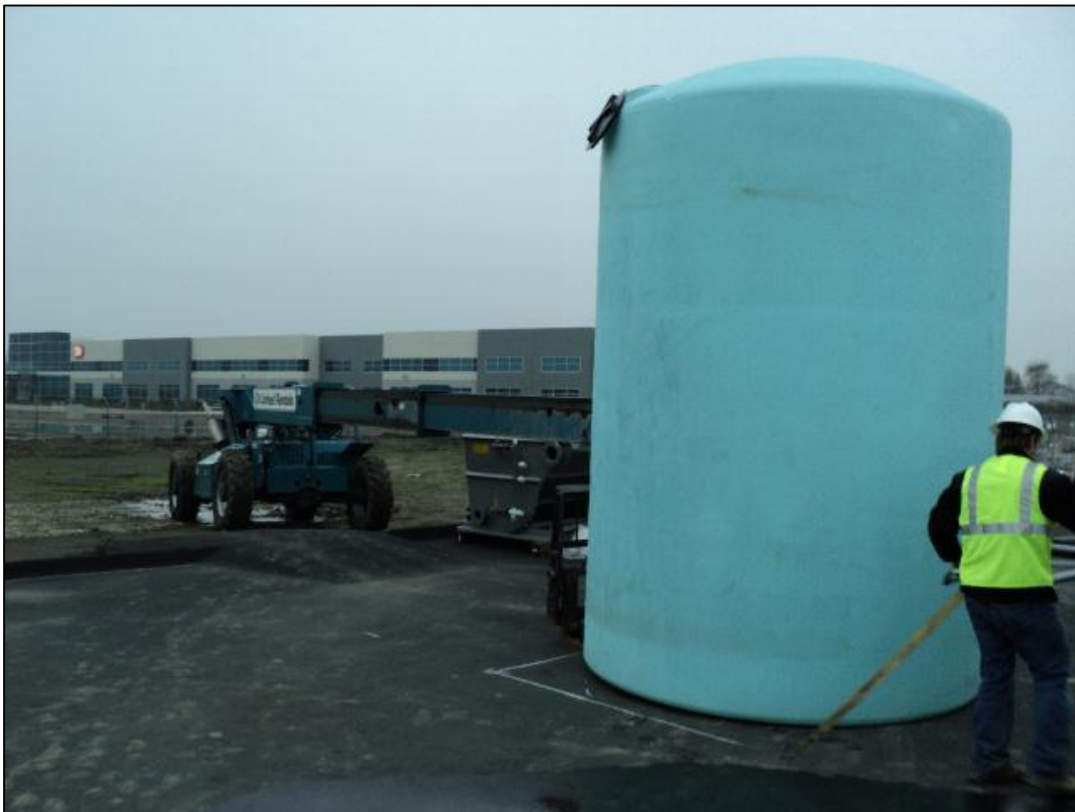
5,000-gallon tank installation.
