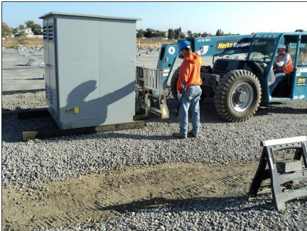
Placement of one of many power transformers at site.
