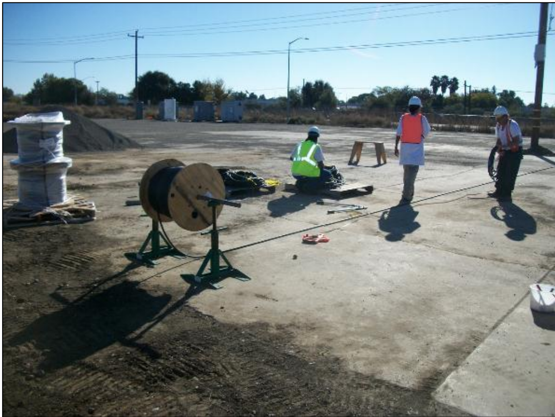
Measurement and cutting of wires.
