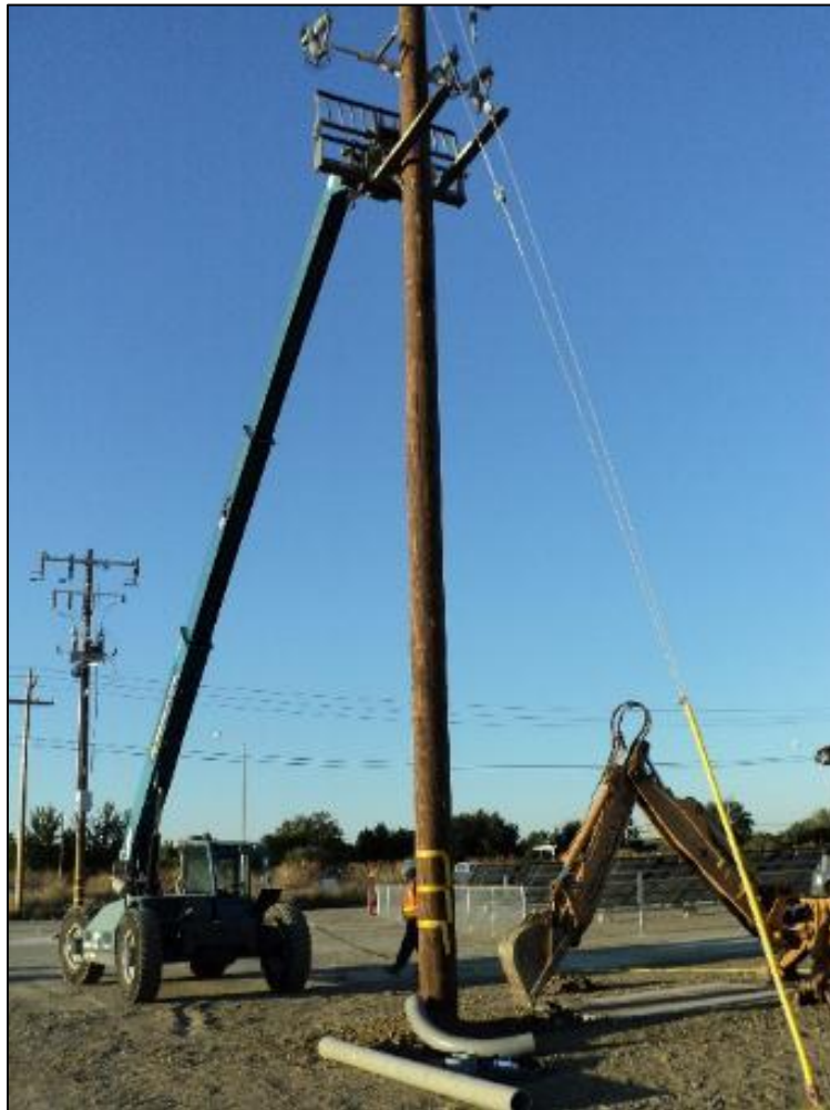
PG&E installing power drop to site transformer.
