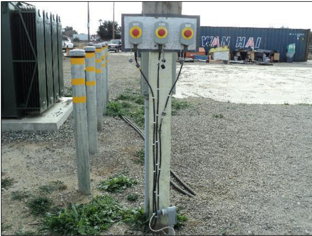
Emergency stop buttons, one per power supply.
