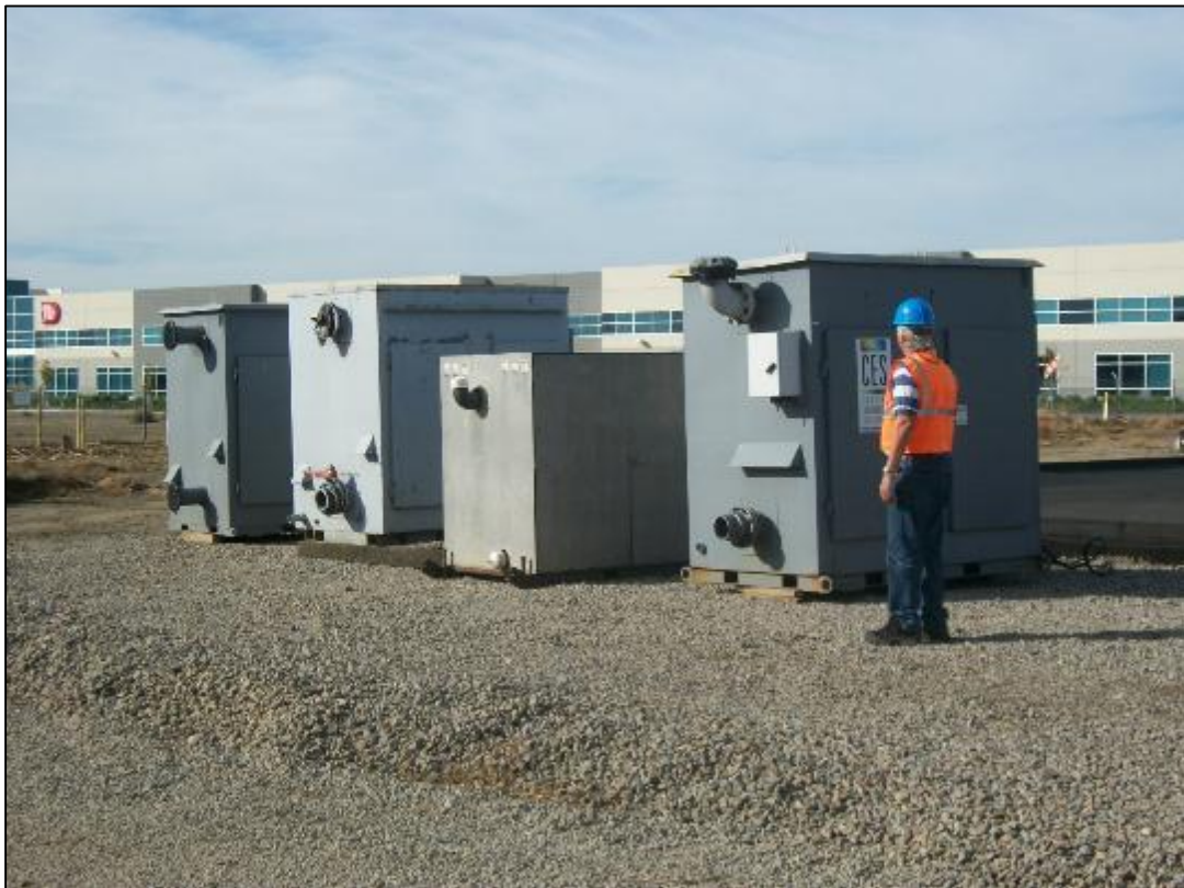
Placement of vacuum extraction units (VEUs). The small unit is the backup blower.
