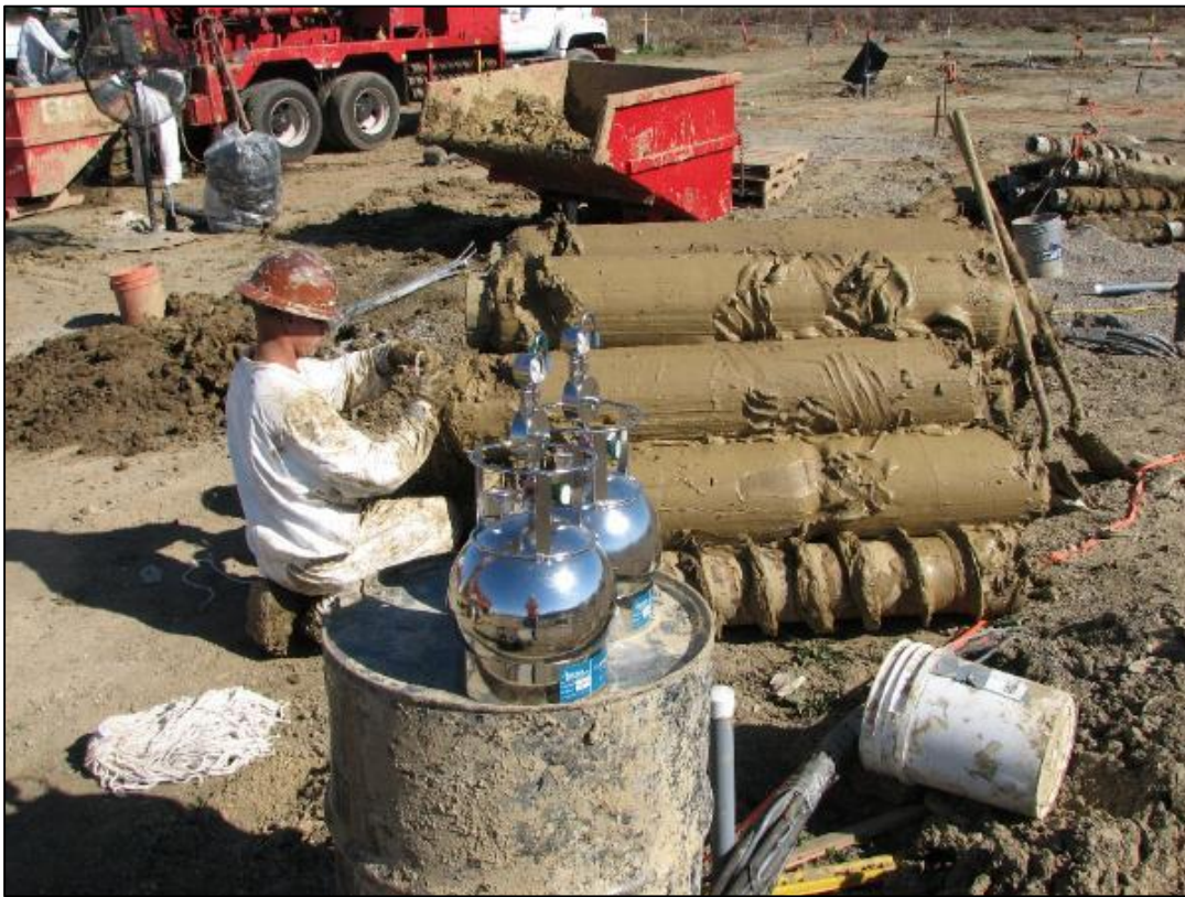
SUMMA canisters used for air monitoring during Installation of electrodes; temperature monitoring wells (TMWs). 2009.
