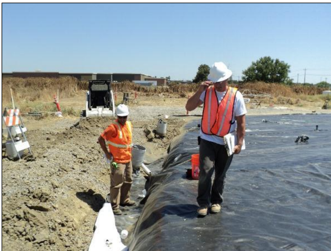
Cap buried at perimeter.
