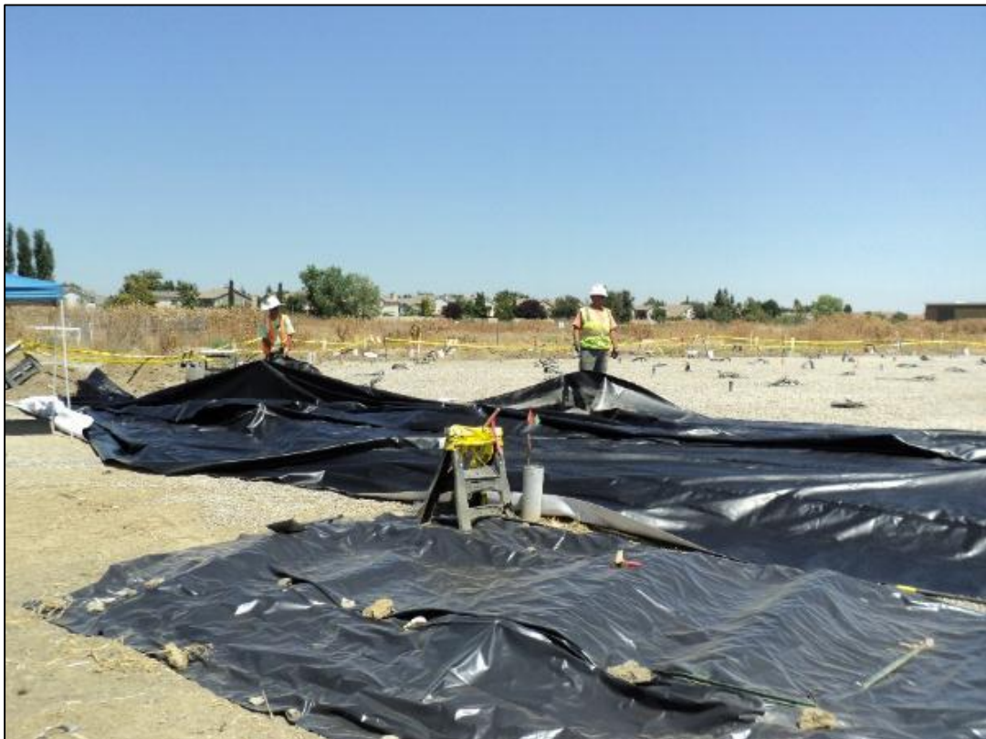
Unfolding layer of high-density polyethylene (HDPE) onto cap.
