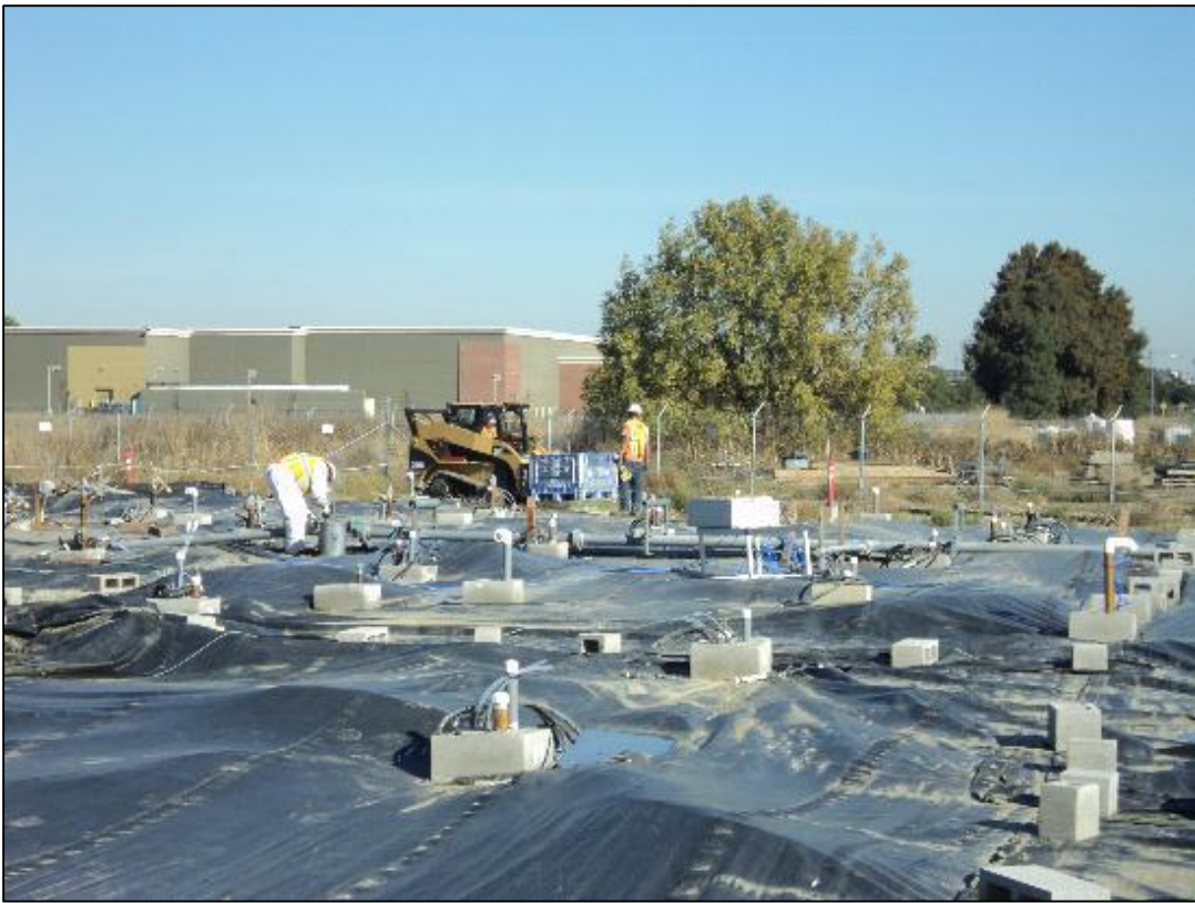
Removal of ISTT components. The lack of wires, manifolds, and skids on the cap is allowing the insulation board to lift significantly.
