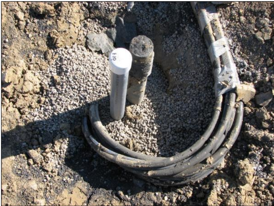
Completed electrode E-10.
