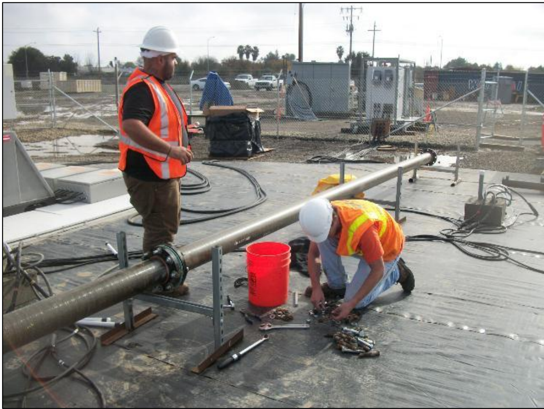
Installing vapor extraction manifold.
