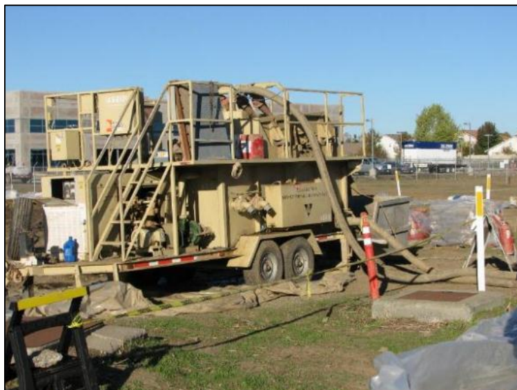
Fluids handling during installation of Preliminary Monitoring Points (PMPs). 2008.
