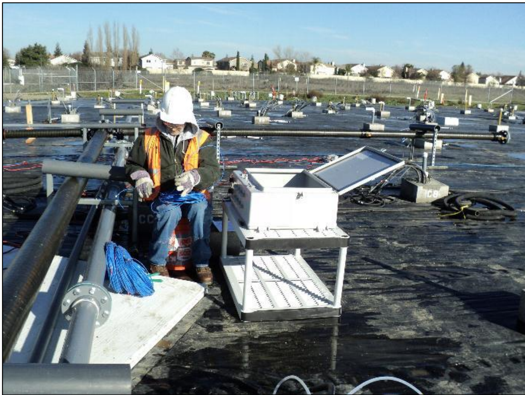
Wiring thermocouples (blue wires).
