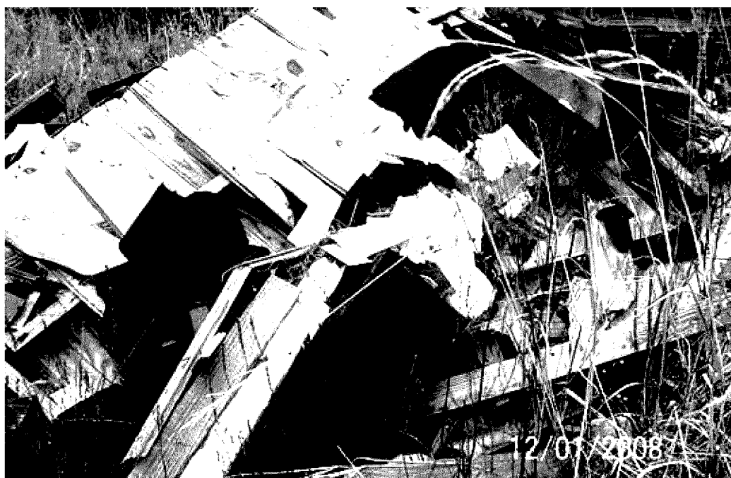
Photo 20: North Property – building debris on northwest portion. Possible asbestos containing material (floor tiles) in this debris pile.
