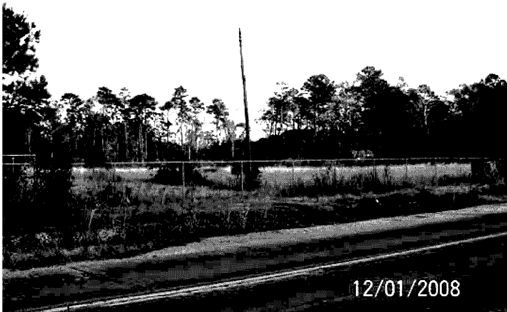
Photo 16: North Property – chain link fence along SH 959
