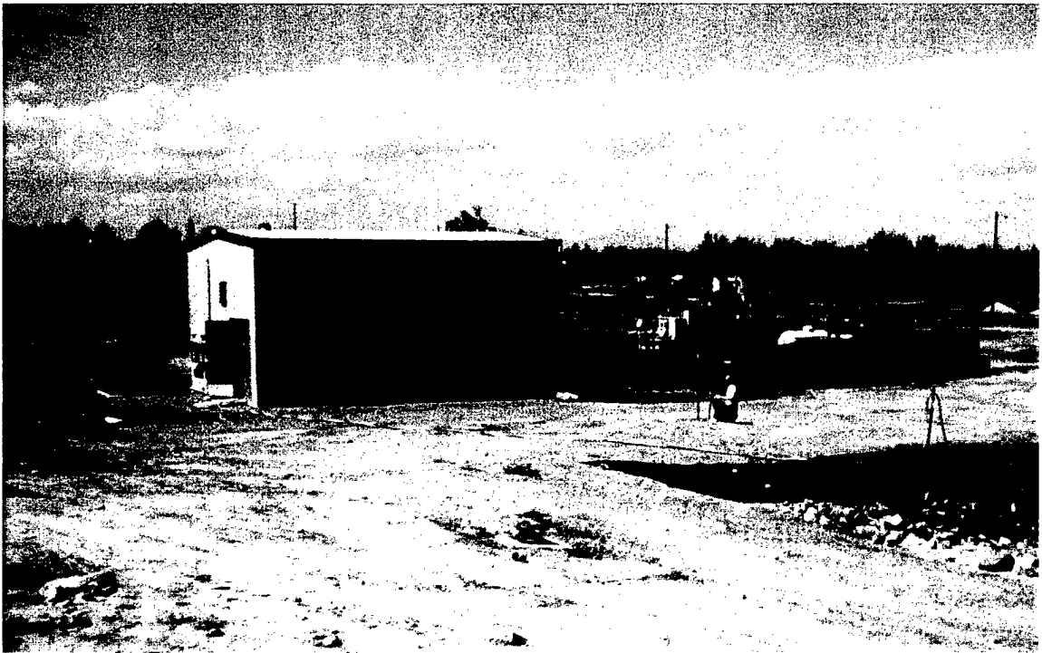
Photograph 1. FTO Treatment System and Source Area Reduction System (SARS) Control Building
