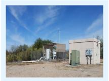
An SVE system with four extraction wells began operating at the Airport Property portion of the Tucson International Airport Area Superfund Site in 2008. The system operates in conjunction with long-term extraction and treatment of groundwater. Vapor-phase GAC adsorbtion is used to treat the extracted vapors. Since SVE startup, optimization has included:
