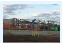
At Site 93 of the Camp Lejeune Military Reservation in North Carolina, a photovoltaic array powers a pump that recirculates contaminated groundwater through a subsurface biogeochemical reactor. Construction of the bioreactor involved injecting 220 gallons of crude soybean oil into a mulch and gravel substrate placed in a 25- by 25-foot cell about 6 feet deep. Approximately 45 cubic yards of uncontaminated excavation soil was used as backfill to minimize import of clean fill.
