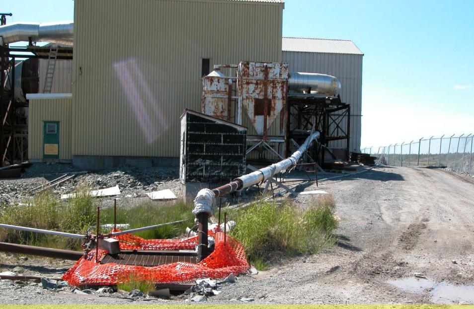
Roasting process to extract gold produced 237,000 tonnes of arsenic dust as byproduct – now in underground storage
