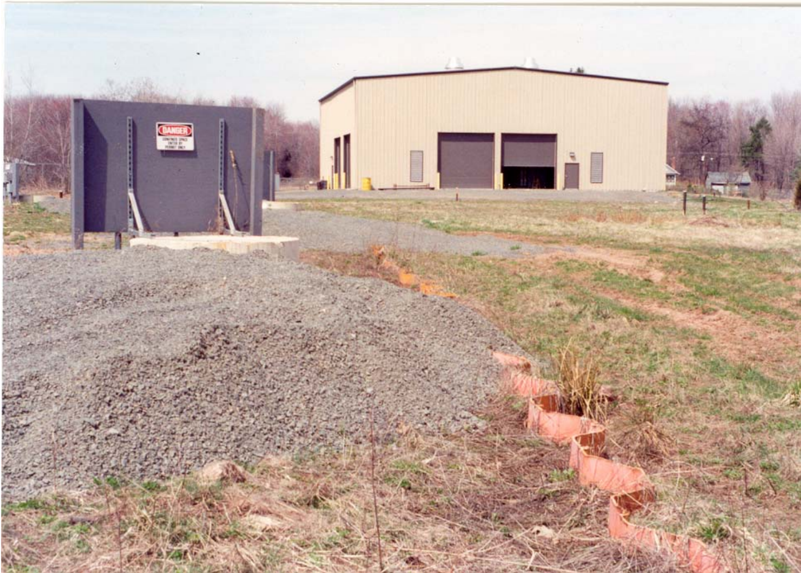
Sheet-pile wall, groundwater recovery well, and the water treatment facility
